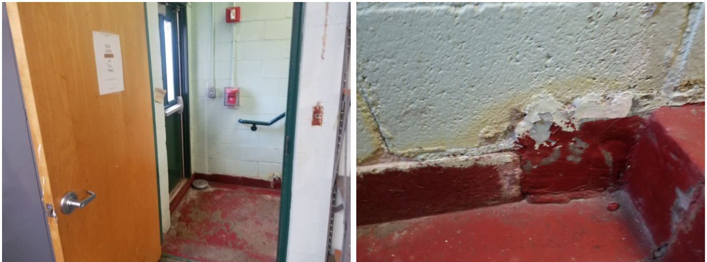
Baldwin School and Soule Recreation Center, Brookline, MA Soule Gymnasium – Basement Stairwell Grout Compound at Wall Intersections (may also contain PCBs)
