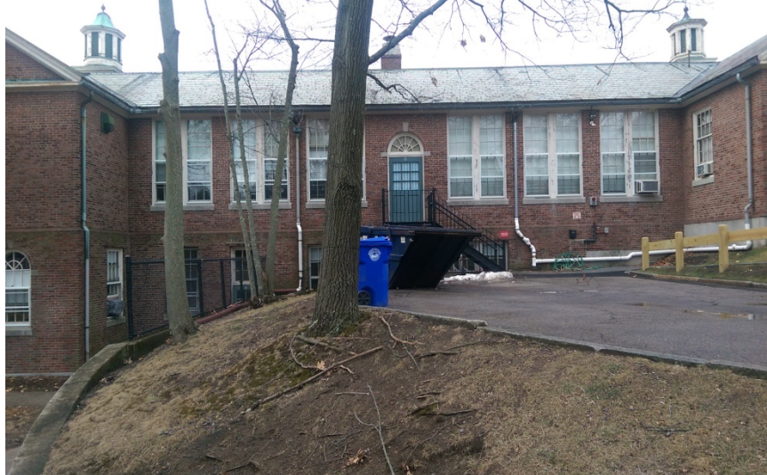
Baldwin School and Soule Recreation Center, Brookline, MA Baldwin School – Exterior Roofing Materials (Shingles, Tar, Sublayers, etc.)
