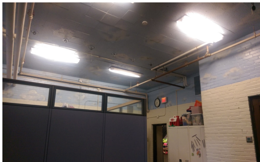
Baldwin School and Soule Recreation Center, Brookline, MA Baldwin School – Basement Activity Room Textured/Cementitious 12"x12" Ceiling Tiles
