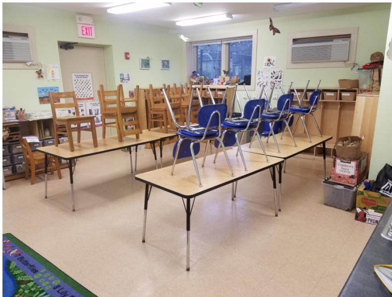
Baldwin School and Soule Recreation Center, Brookline, MA Soule Environmental Education Center – RM1 Tan Flooring and Wallboard & Joint Compound (on ceilings and walls)
