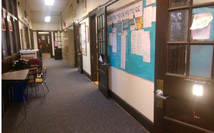
Baldwin School and Soule Recreation Center, Brookline, MA Baldwin School – 1 st Floor Hallway Blue Carpet w/ Mastic
