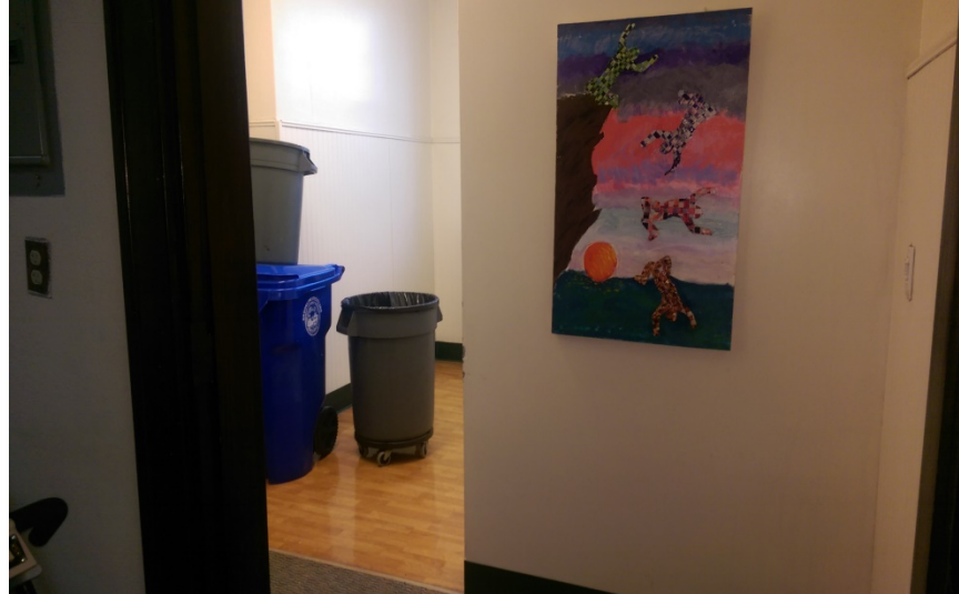
Baldwin School and Soule Recreation Center, Brookline, MA Baldwin School – 1 st Floor Bathroom Wainscoting w/ Mastic on Plaster Walls
