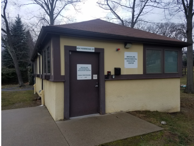
Baldwin School and Soule Recreation Center, Brookline, MA Soule Environmental Education Center – 654 Hammond Street
