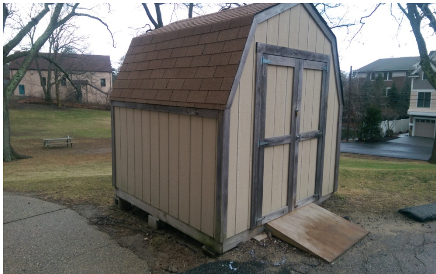
Baldwin School and Soule Recreation Center, Brookline, MA Baldwin School – Exterior Storage Sheds Roofing Material (Shingles, Tar, Sublayers, etc.)
