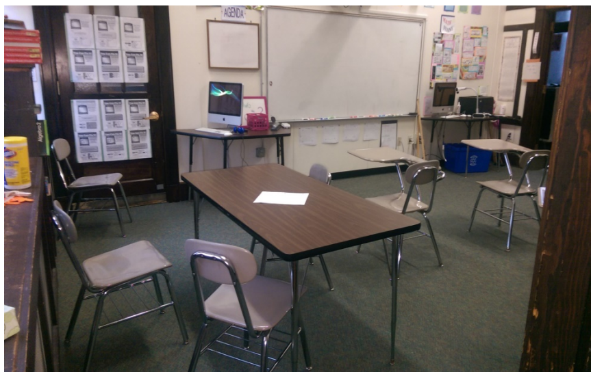
Baldwin School and Soule Recreation Center, Brookline, MA Baldwin School – 1 st Floor Classrooms and Offices Green Carpet w/ Mastic
