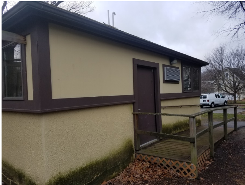
Baldwin School and Soule Recreation Center, Brookline, MA Soule Environmental Education Center – Exterior Stucco/Cementitious Siding Material
