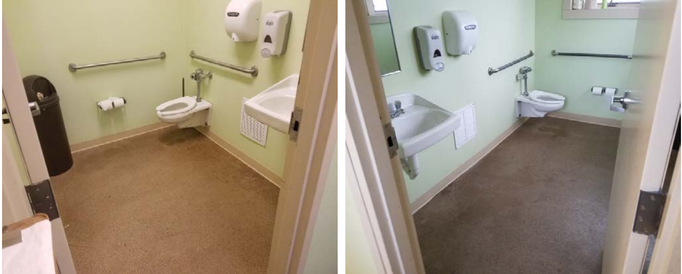
Baldwin School and Soule Recreation Center, Brookline, MA Soule Environmental Education Center – RM2 (left) and RM3 (right) Tan Flooring w/ Mastic, Tan Cove Base w/ Mastic, and Light-green Wallboard and Joint Compound.
