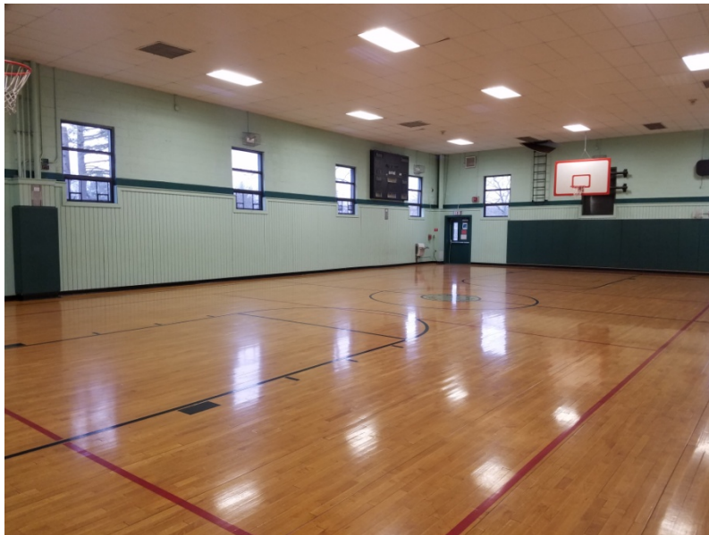
Baldwin School and Soule Recreation Center, Brookline, MA Soule Gymnasium – RM5 Black Cove Base w/ Mastic and White 2' x4' Acoustical Ceiling Panels
