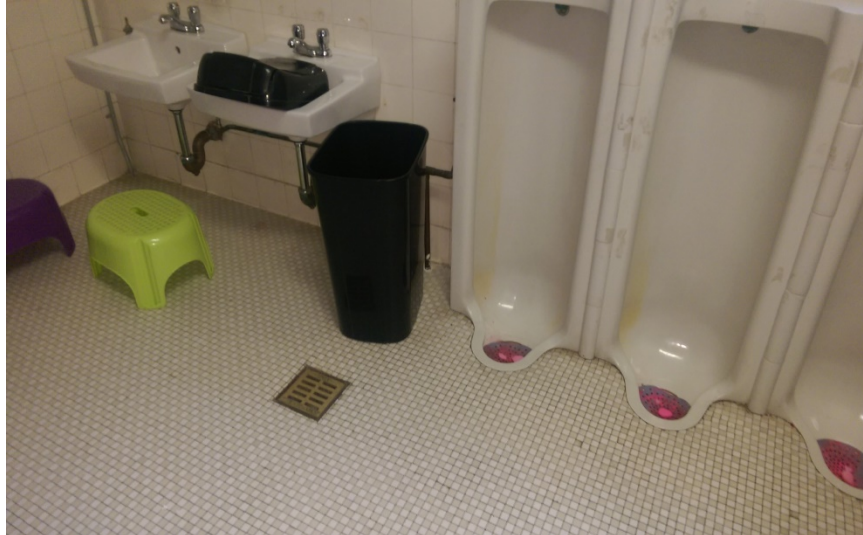
Baldwin School and Soule Recreation Center, Brookline, MA Baldwin School – Bathrooms on 1 st Floor ½” White Floor Tile w/ Grout & Mastic
