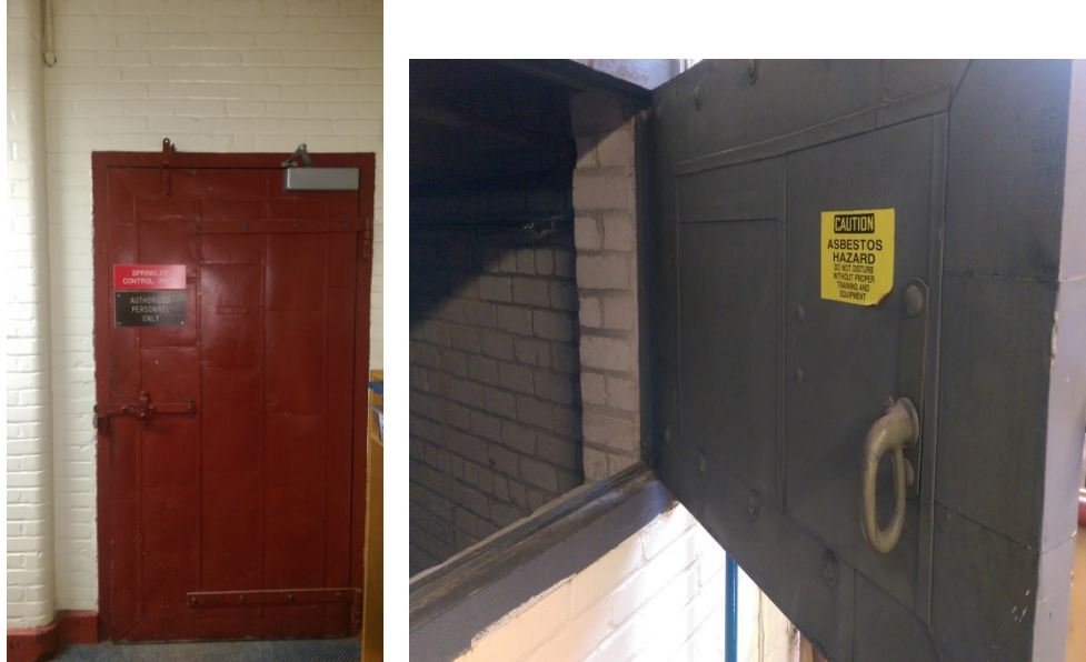
Baldwin School and Soule Recreation Center, Brookline, MA Baldwin School – Boiler Room Fire Safe Doors
