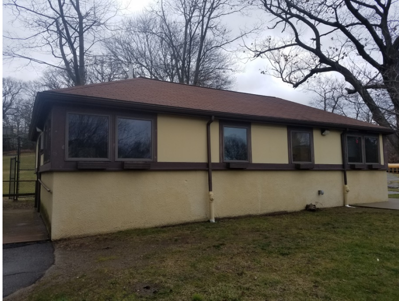
Baldwin School and Soule Recreation Center, Brookline, MA Soule Environmental Education Center – Exterior Roofing Material (Shingles, Tar, Sublayers, etc.)
