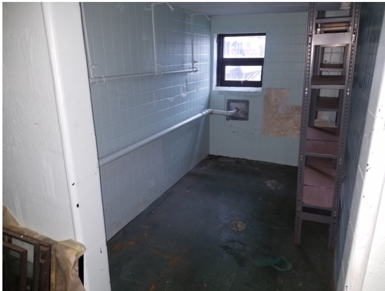
Baldwin School and Soule Recreation Center, Brookline, MA Soule Gymnasium – RM2 (Basement) Blue Wall Tile w/ Grout & Mastic and Black Floor Tile w/ Grout & Mastic
