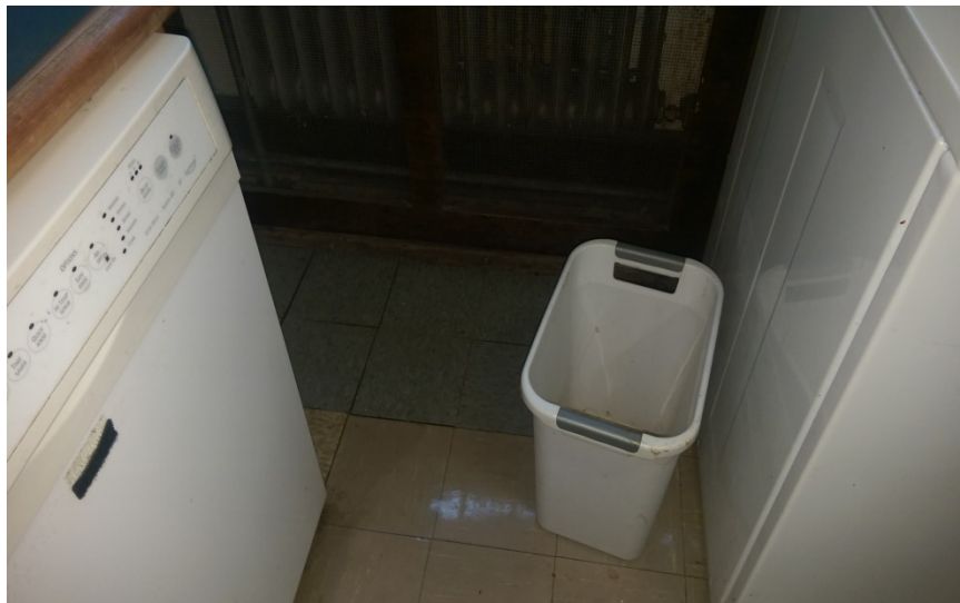
Baldwin School and Soule Recreation Center, Brookline, MA Baldwin School – Kitchen Green 9"x9" Floor Tiles w/ Mastic
