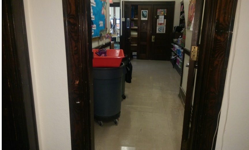
Baldwin School and Soule Recreation Center, Brookline, MA Baldwin School – Kitchen, and under carpet in Classroom/Lunchroom, and Lounge Tan 9"x9" Floor Tiles w/ Mastic
