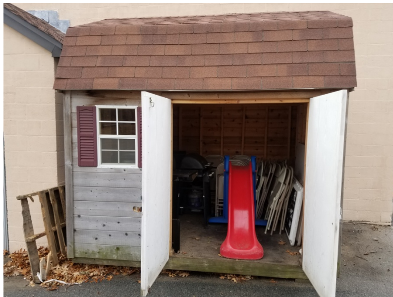
Baldwin School and Soule Recreation Center, Brookline, MA Soule Gymnasium – Exterior Storage Shed Roofing Materials
