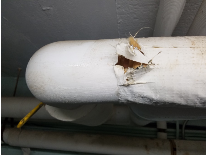
Baldwin School and Soule Recreation Center, Brookline, MA Soule Gymnasium – Attic, behind Walls/Ceilings Pipe Fitting Insulation on Fiberglass-insulated Pipes (joints and elbows)
