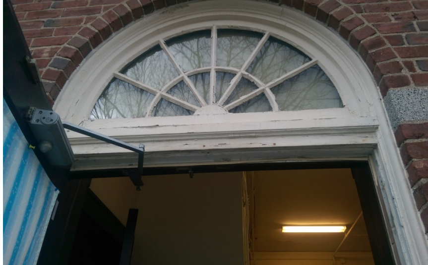
Baldwin School and Soule Recreation Center, Brookline, MA Baldwin School – Exterior Window Glazing and Caulking (may also contain PCBs)
