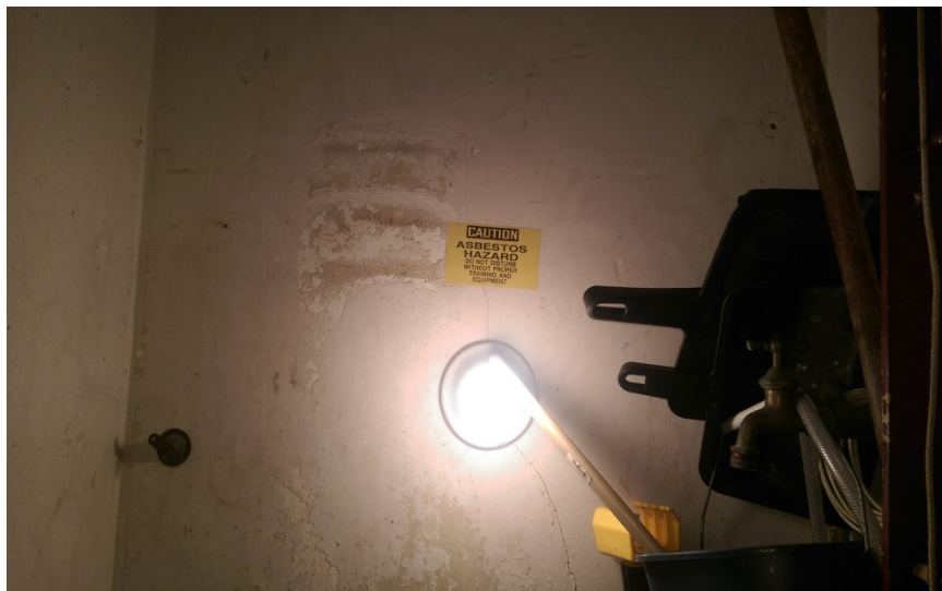
Baldwin School and Soule Recreation Center, Brookline, MA Baldwin School – Throughout (classrooms, bathrooms, office/storage, and hallways) Smooth Plaster on Ceilings and Walls
