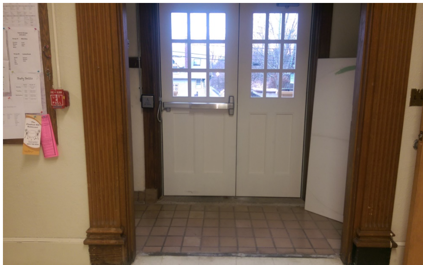
Baldwin School and Soule Recreation Center, Brookline, MA Baldwin School – Front and Side Entrances Red/Brown 4"x4" Floor Tiles w/ Grout & Mastic
