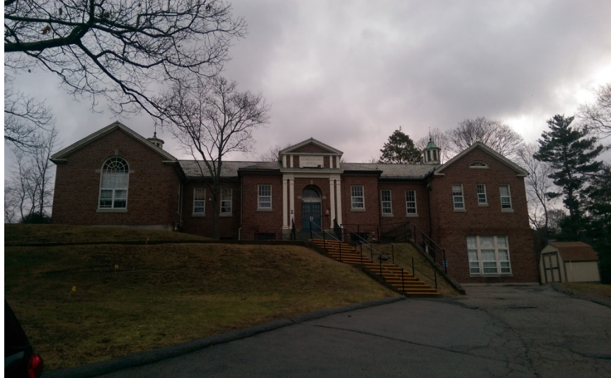
Baldwin School and Soule Recreation Center, Brookline, MA Baldwin School – 484/490 Heath Street
