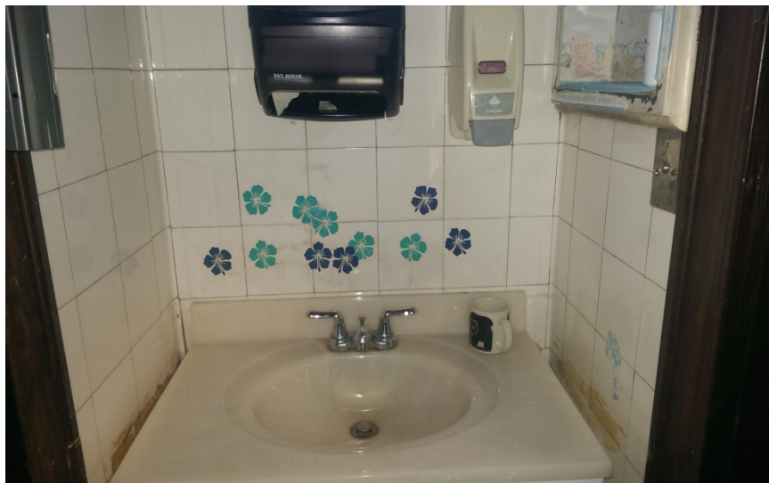
Baldwin School and Soule Recreation Center, Brookline, MA Baldwin School – Bathrooms and Water Fountain Areas on 1 st Floor Wall Tile w/ Grout & Mastic
