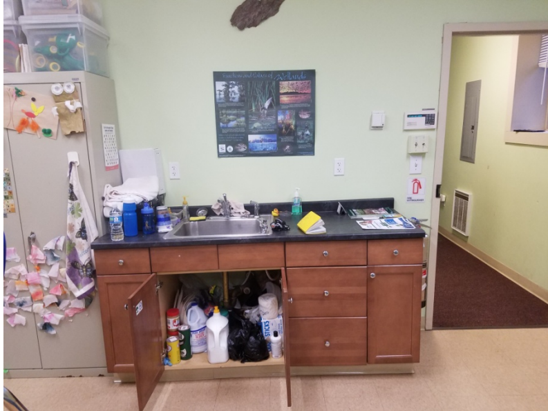
Baldwin School and Soule Recreation Center, Brookline, MA Soule Environmental Education Center – RM1 Tan Cove Base w/ Mastic, and Black Laboratory Counter Top
