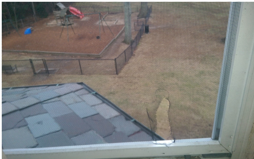
Baldwin School and Soule Recreation Center, Brookline, MA Baldwin School – Exterior Roofing Material (Adhesive on Clay/Slate Shingles, Tar, Sublayers, etc.)
