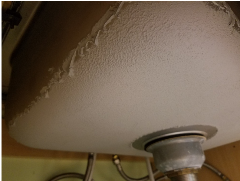
Baldwin School and Soule Recreation Center, Brookline, MA Soule Environmental Education Center – RM1 White Textured Insulation on Underside of Sink.
