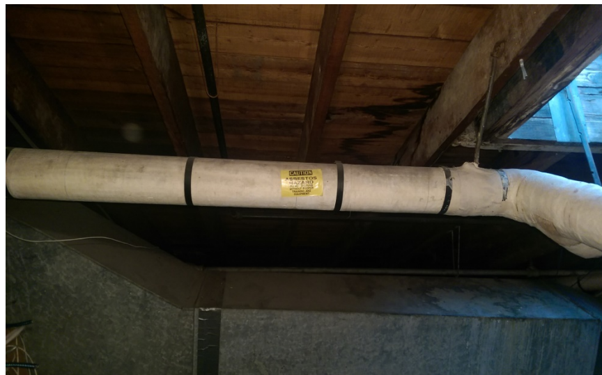
Baldwin School and Soule Recreation Center, Brookline, MA Baldwin School – Attic, Boiler Room, and behind Walls/Ceilings Pipe Fitting Insulation on Fiberglass-insulated Pipes (joints and elbows)
