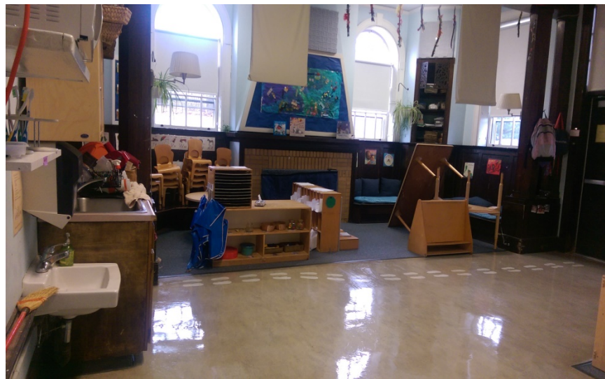
Baldwin School and Soule Recreation Center, Brookline, MA Baldwin School – Basement Classrooms, Nap Room, Bathroom, and Hallway Tan Flooring w/ Mastic
